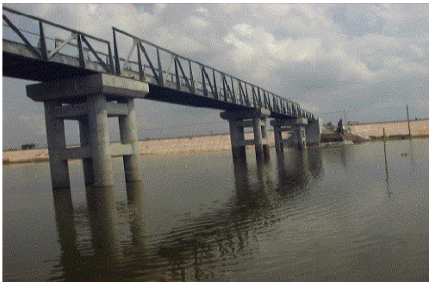
Photo 3 Newly constructed 100 m bridge in place of damaged 67 m bridge (After: Haque et al., 2002)
